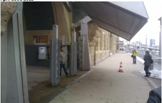
Photo: Flood barrier in the low-lying part of the city of Hamburg, Germany. Flood proofing of urbanised areas is a good option at the local scale but not for large areas.
